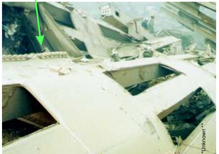
Figure 3-11 The bolts holding the pre-fab units together.
