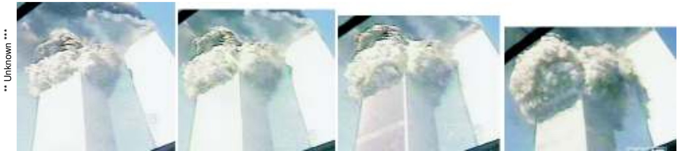
Figure 7-11 Four frames of video show the collapse progressed floor by floor in a nearly perfectly balanced manner.
